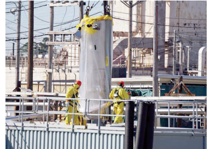
SRR employees install an ion-exchange column.
